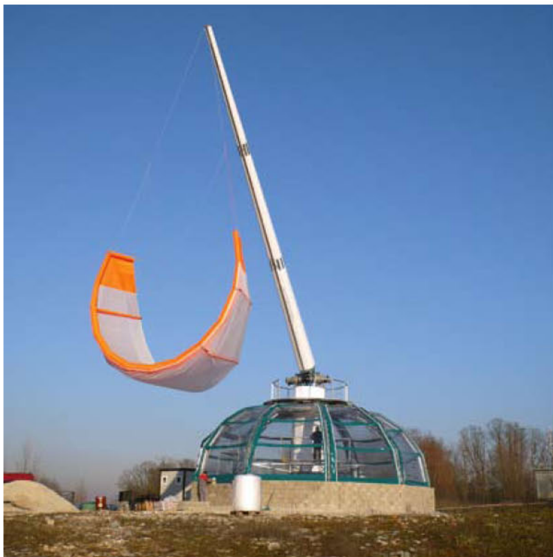
The kite-driven power plant from Kite Gen achieves an output of up to 3 MW – here a prototype which went into operation in 2011.
